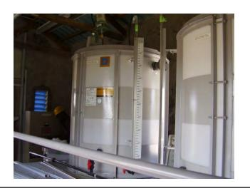
Chlorine Solution Tank Volume: 1,000L
