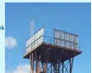
196m3 Elevated Tank Rehab in Kasama
