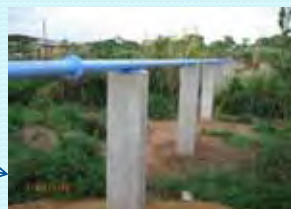
Distribution network rehab in Kasama
