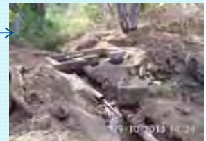
Kasoka Intake -Before
