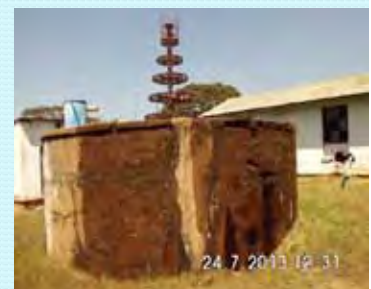
Mbala District – Existing water treatment Tank at Chila Plant
