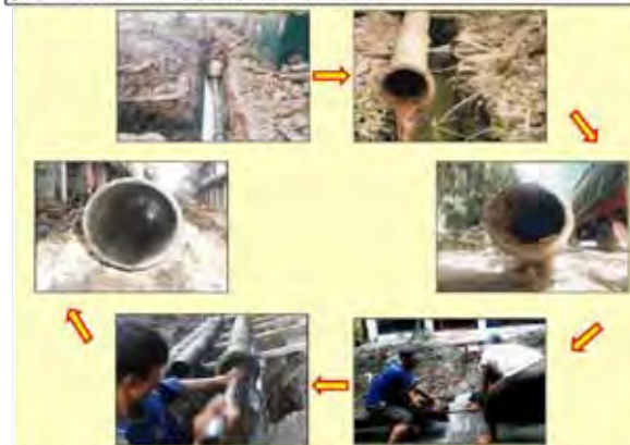
(1-2) PIPE LINE CLEANING AND REINSTALLATION
