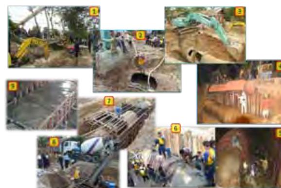
(1-4) TRANSMISSION PIPE BURST REPAIRMENT
