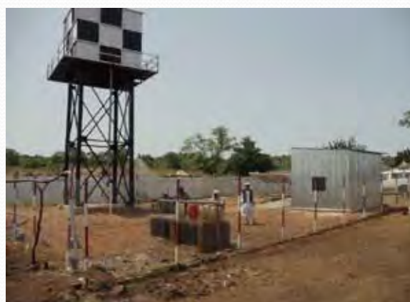
Al - Gari Water Yard
