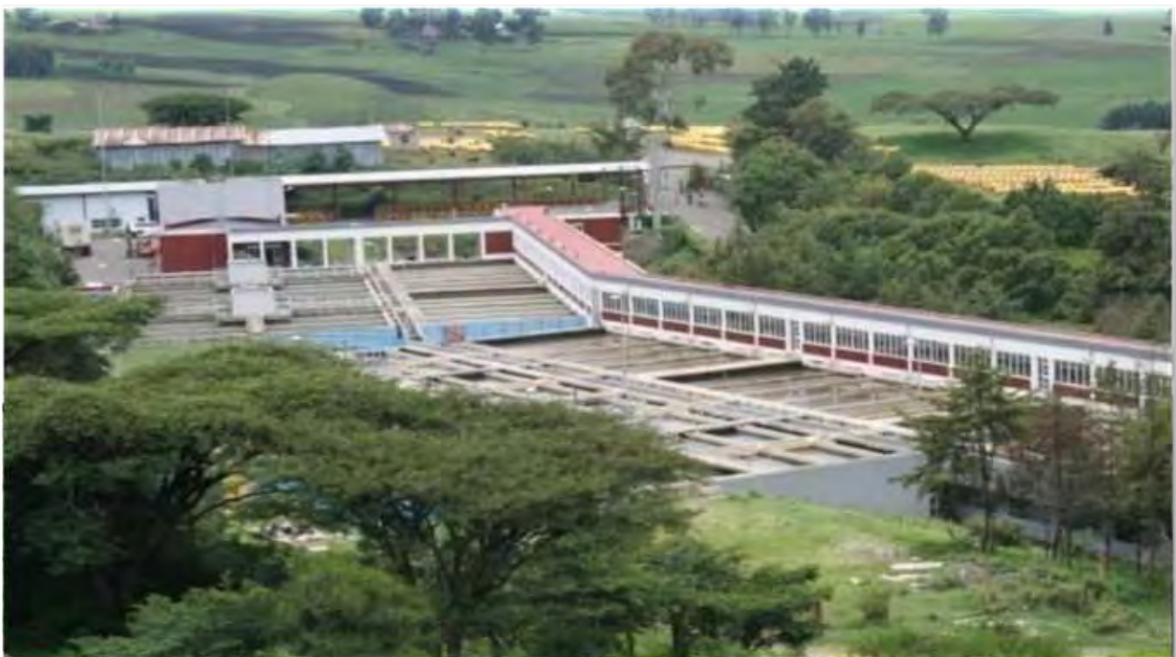
Picture: Legedadi water treatment plant
