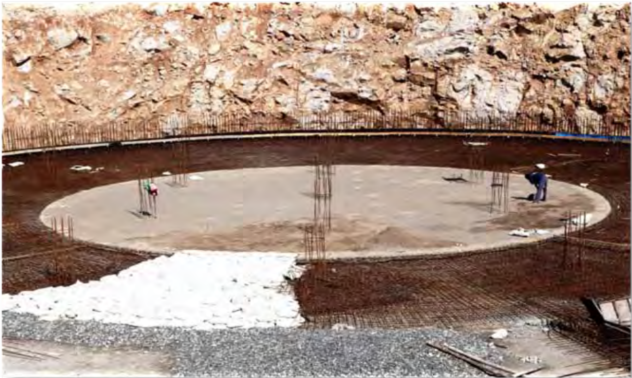
Picture: Construction of reservoir in Hanamariam area
