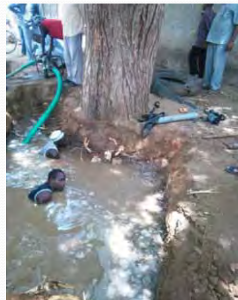
Blockage of water pipelines with trees roots
