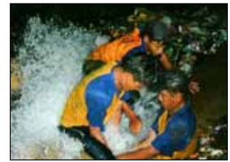
Frequent Pipe Break in Transmission line
