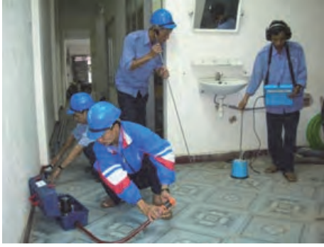
No 5. Leakage Detecting in household
