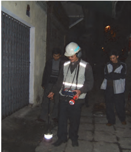
No 6. Leakage Detecting on street
