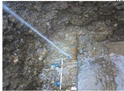
No3. Joint leaking
