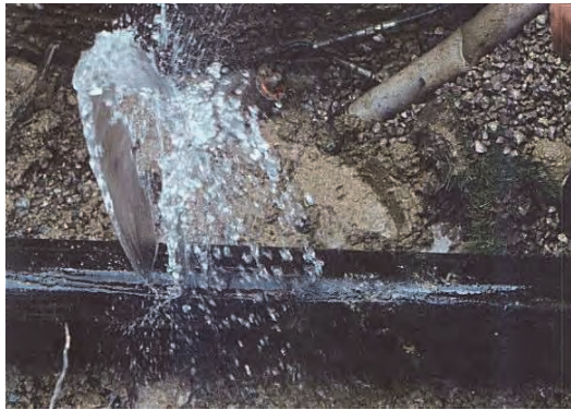
No1. Pipe cracking
