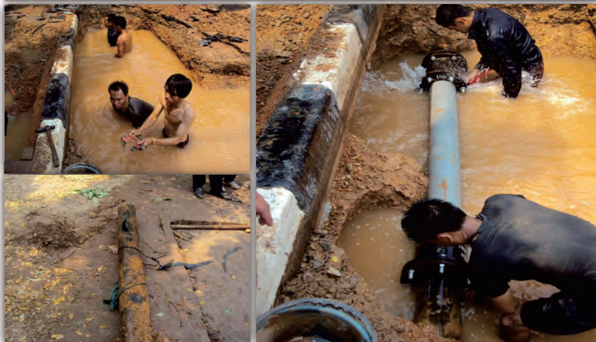
Leakage on transmission pipe SP 150mm under asphalt road
