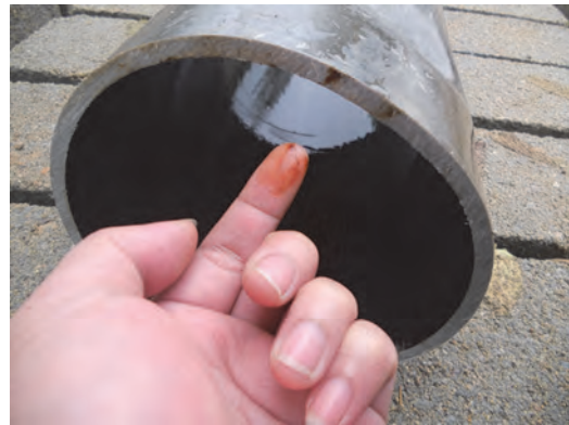
No4. Rust inside the pipe
