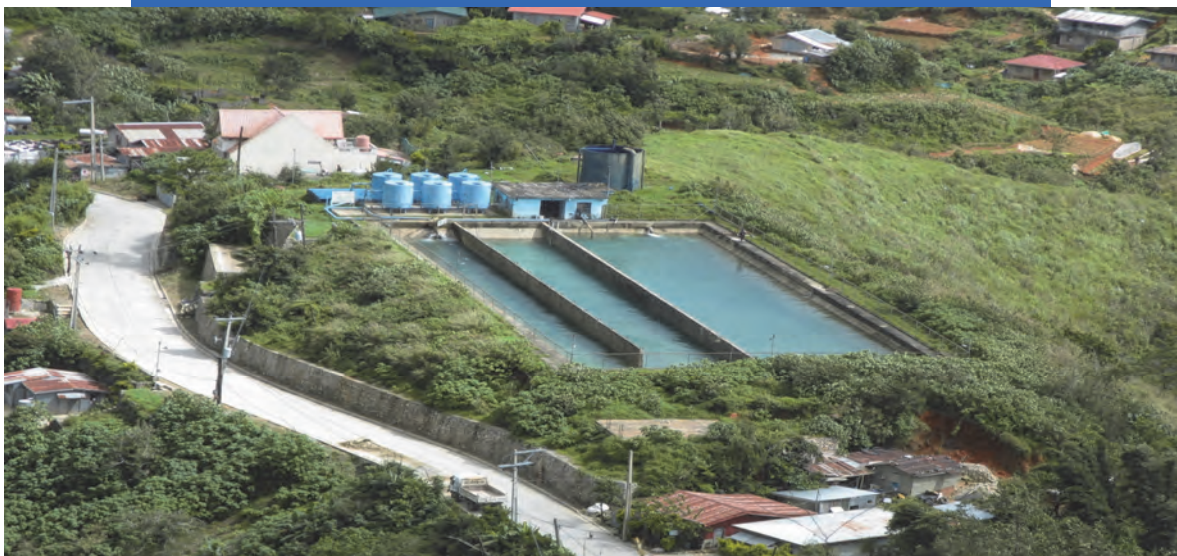
Km 8 reservoir and water treatment plant; Capacity: 5,687 cu.m.
