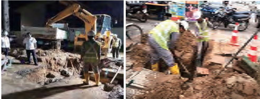
Water Leakage Repairing
