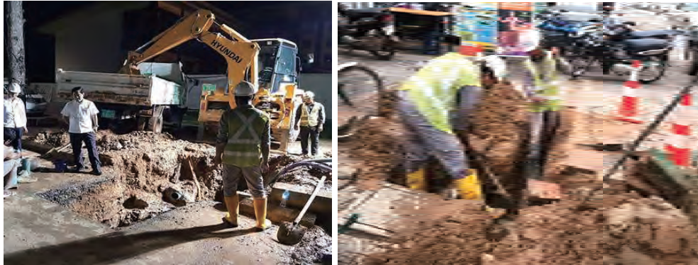
Water Leakage Repairing
