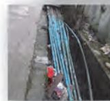
Aged Transmission Pipes in Yangon City Water Supply System
