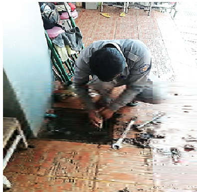
Repairing House Service Water Meter
