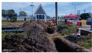
Trenching and pipe installation at Culvert #6, CH 2+620m
