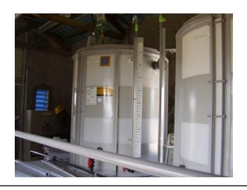
Chlorine Solution Tank Volume: 1,000L
