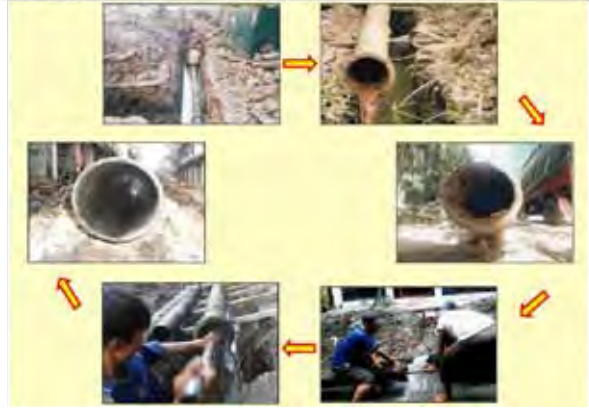
(1-4) TRANSMISSION PIPE BURST REPAIRMENT
