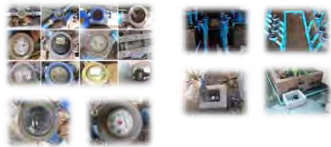
1-3) DAMAGED METER REPLACEMENT AND NEW METER INSTALLATION
