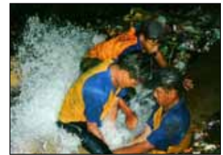
Frequent Pipe Break in Transmission line
